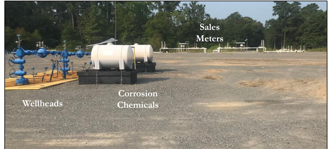
Typical full well stream wellsite
